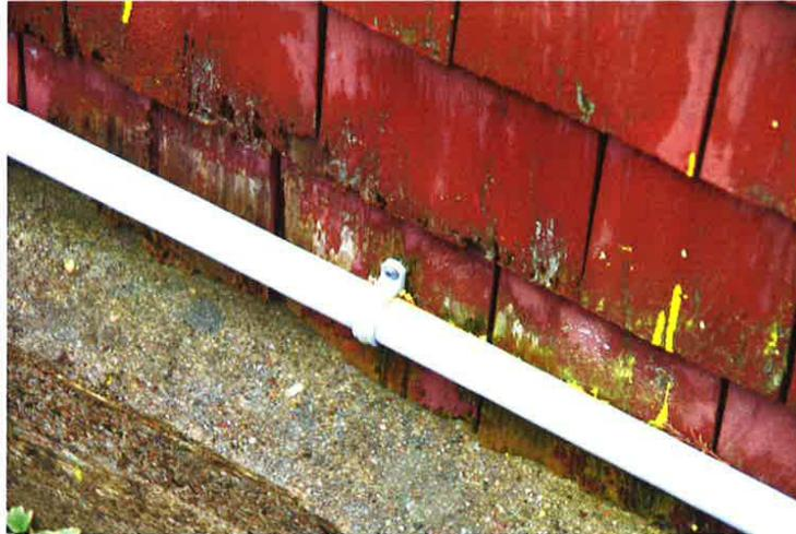
Photo 11: Typical condition of siding near foundation level.
