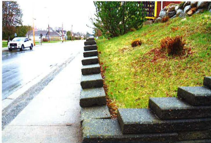
Photo 4: Interlocking block retaining wall.
