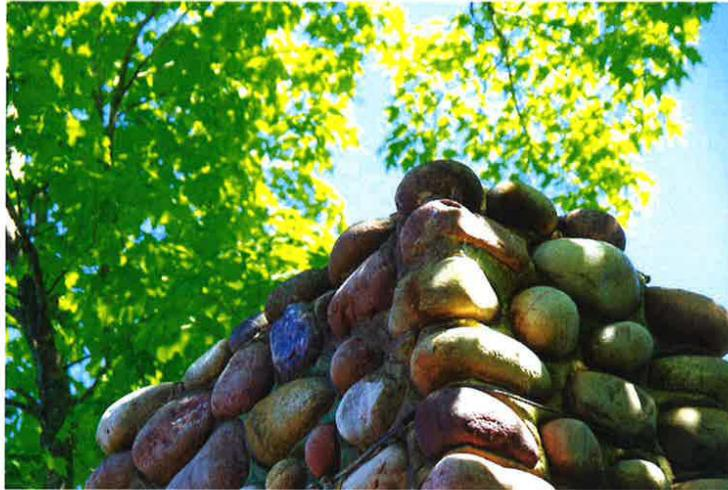
Photo 9: Top of stone chimney. Note lack of rain cap and steel cable wrap.
