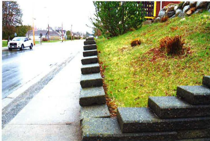
Photo 4: Interlocking block retaining wall.
