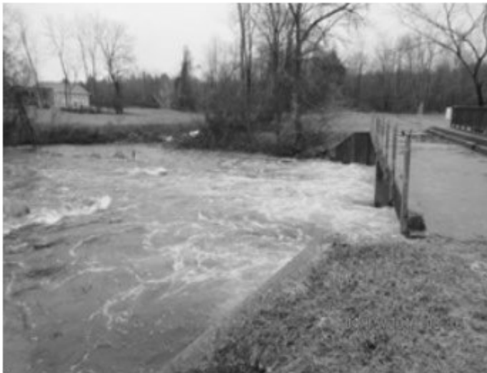
Photo 55 Downstream View of Bennett Dam
