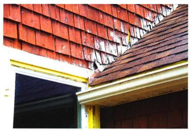
Photo 10: Roof wall interface at rear of south addition. Note siding deteriorated.
