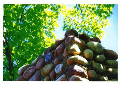
Photo 9: Top of stone chimney. Note lack of rain cap and steel cable wrap.
