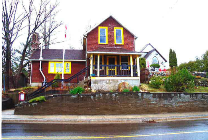
Photo 1: Building viewed from street. East elevation.
