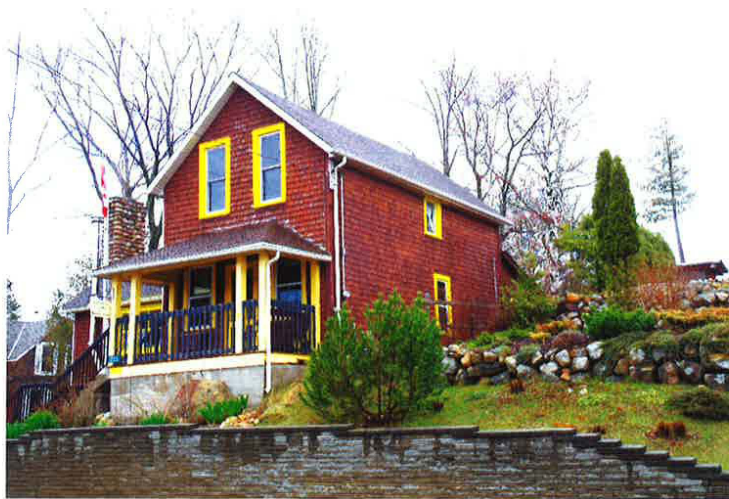
Photo 2: Building viewed from street. North elevation
