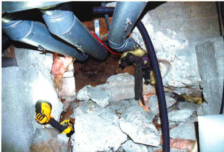
Photo 12: Opening from basement to crawlspace.
