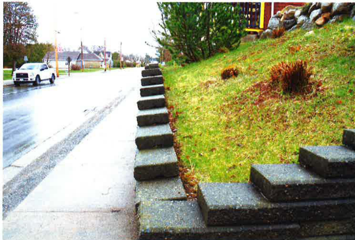
Photo 4: Interlocking block retaining wall.
