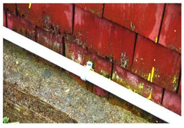
Photo 11: Typical condition of siding near foundation level.
