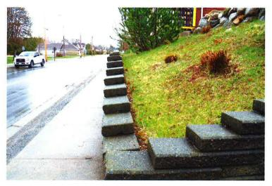
Photo 4: Interlocking block retaining wall.
